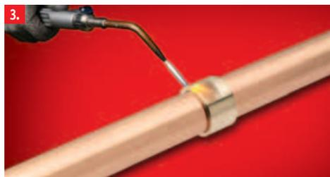
If the complete ring of solder does not appear on heating, apply additional flux to the mouth of the socket and end feed the joint with our N165 or N166 cadmium-free silver brazing alloy, or an equivalent to the compositional requirements of BS EN 1044 AG103 (formerly BS 1845 AG14).
